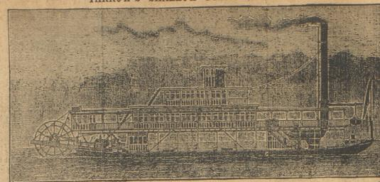
ERNWHEEL STEAMERS have been found by experience to be the best type of vessel for shallow river navigation, and of these Messrs. Yangow have constructed a large number of successful examples for all parts of the world.
