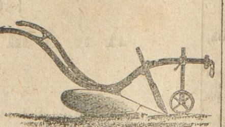
This is one of the smallest Ploughs made by J. & F. HOWARD. It is suitable for a small mule or pony, and is adapted for stirring loose soil and for any kind of shallow ploughing, where the draught is light.
