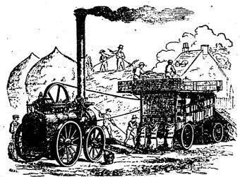
This Engraving shows one of RUSTON, PROCTOR, and CO.'S celebrated PORTABLE STEAM ENGINES, and combined PATENT THRASHING and FINISHING DRESSING MACHINES, as in work, Thrashing and preparing the Corn for Market at one
