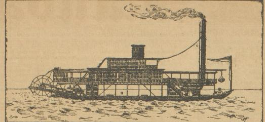
TERNWHEEL STEAMERS have been found by experience to be the best type of vessel for shallow river navigation, and of these Messrs. Yankow have constructed a large number of successful examples for all parts of the world. Vessels on this system are constructed when required, to draw as little as 6 inches.
